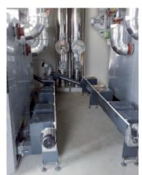
This image shows the ash container of a 2 HERZ boiler cascade solution connected via the screw system.
